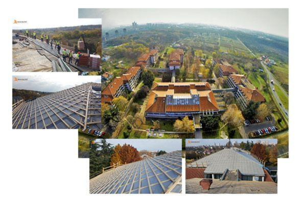
The Gerontological Center 'Bežanija' hired us for the needs of roof repairing which included setting up new wooden beams, installing thermal insulation and replacing old and worn roof tiles with new ones.
