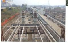
North Approach Roads of Bridge over the river Sava; LOT 2 (from New Belgrade Railway Station to Jurij Gagarin Interchange) is approximately 1km long comprising 2×1000 m elevated, three lane, dual carriageway and 1000 m two track viaduct for the future Belgrade Metro (BGM).
